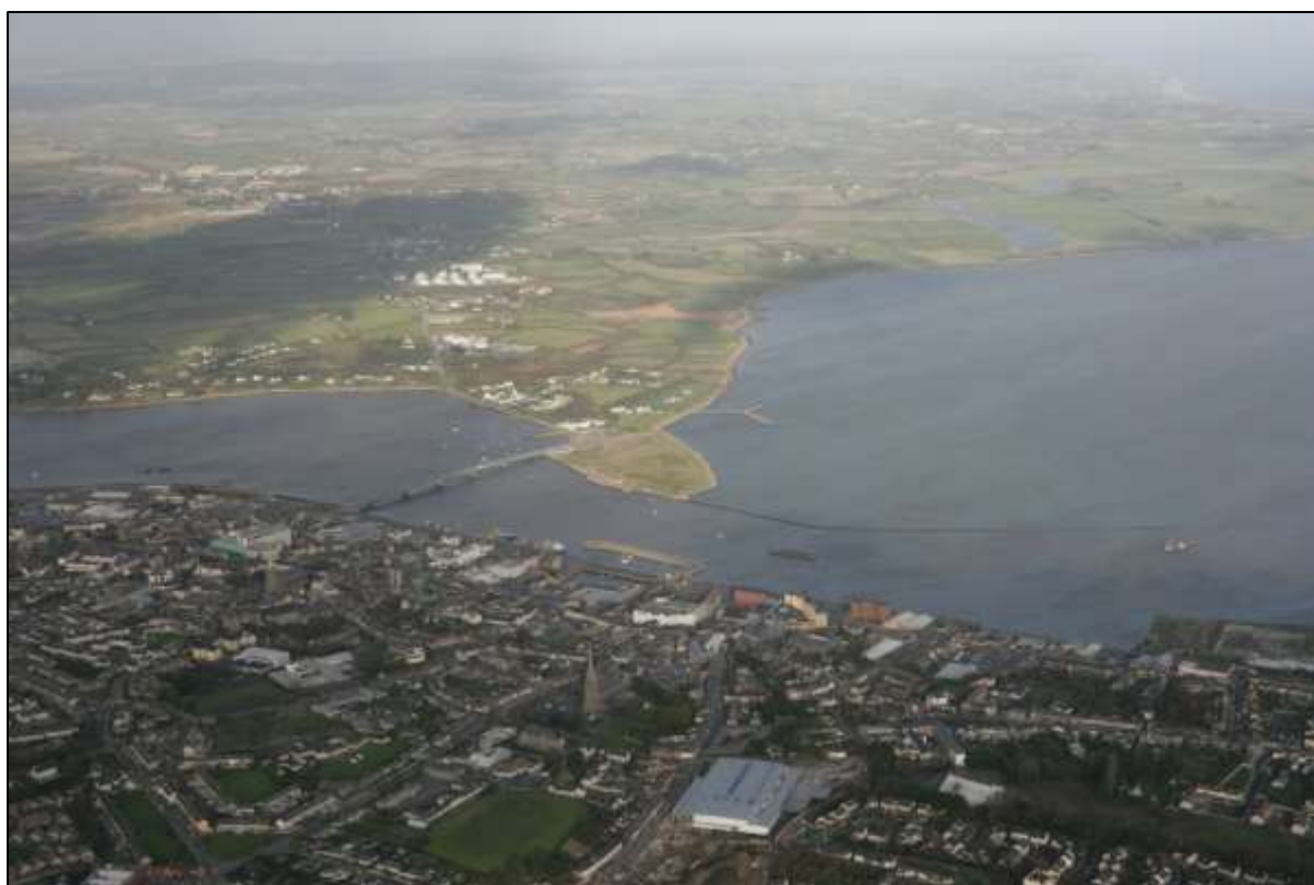
Plate 3.2. Aerial photo of the Lower Slaney Estuary at Wexford Harbour. (Photo courtesy of IFI and No. 3 Operational Wing, Irish Air Corps [Aer Chór na hÉireann])
