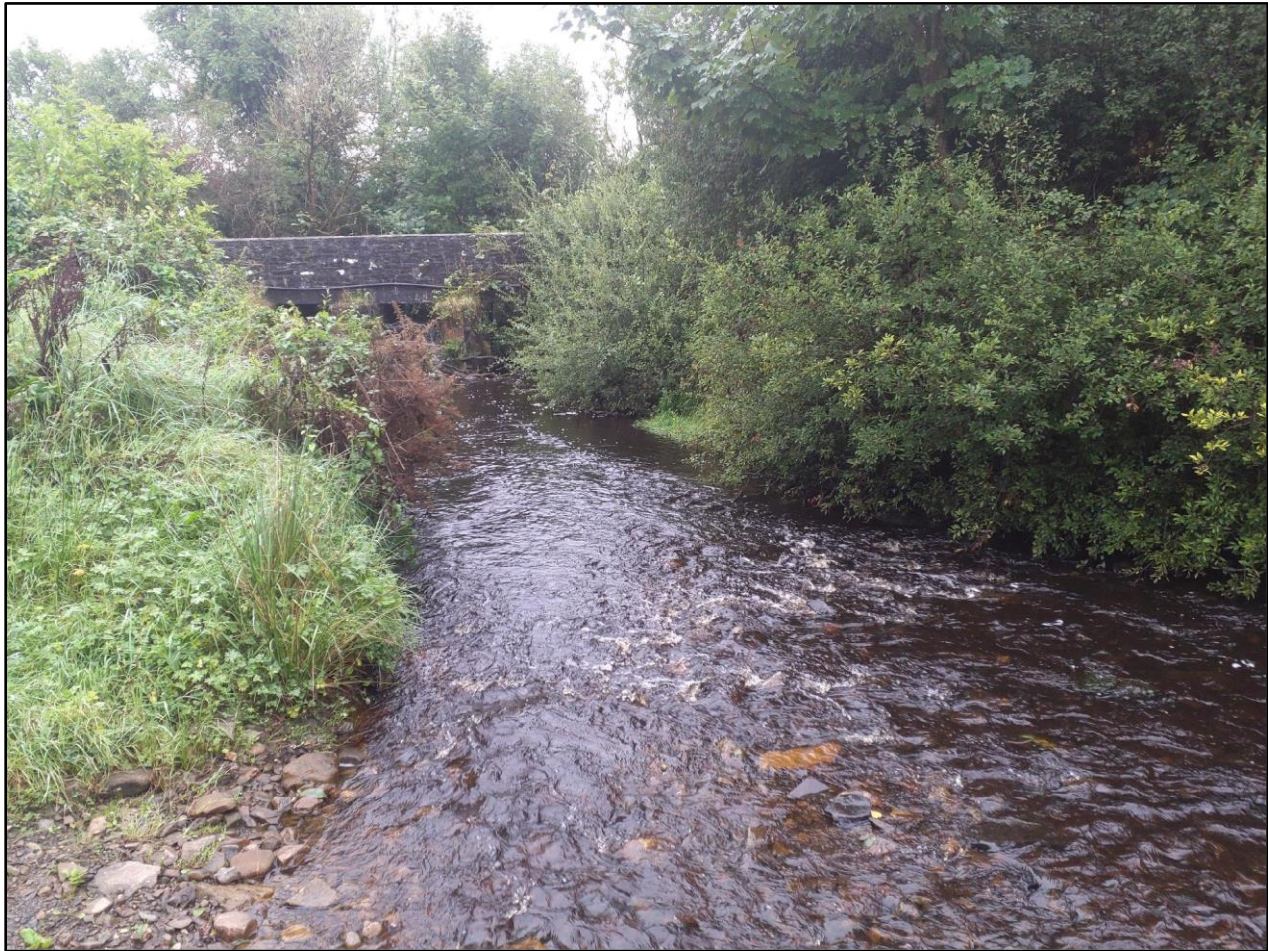
The Cloghboola River at Glena Bridge, Owveg sub-catchment (Site 18).
